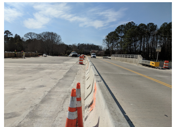
An eastbound view of the Lakeview Road Direct Connector bridge
