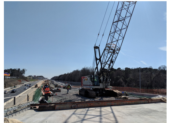
Crews constructing the Hambright Direct Connector bridge deck
