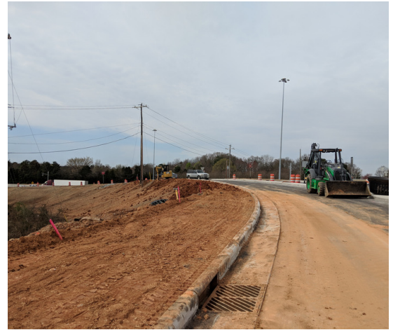
Crews constructing the sidewalk at Exit 30/Griffith Street
