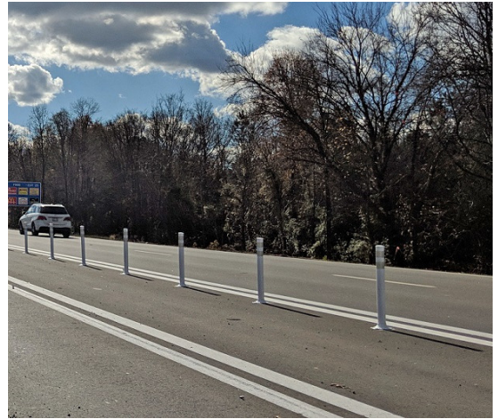
Lane delineator installation
