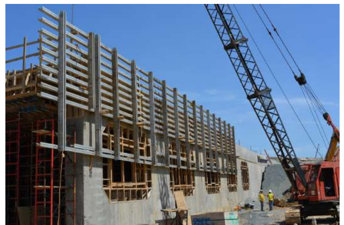
Forming the roof slab at the new Express Lanes underpass just north of the I-85/I-77 interchange.
