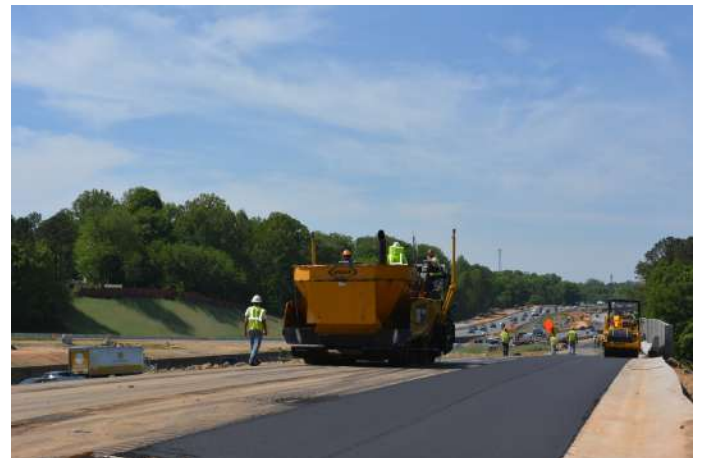
Paving the northbound on-ramp at Exit 12 LaSalle Street in Charlotte
