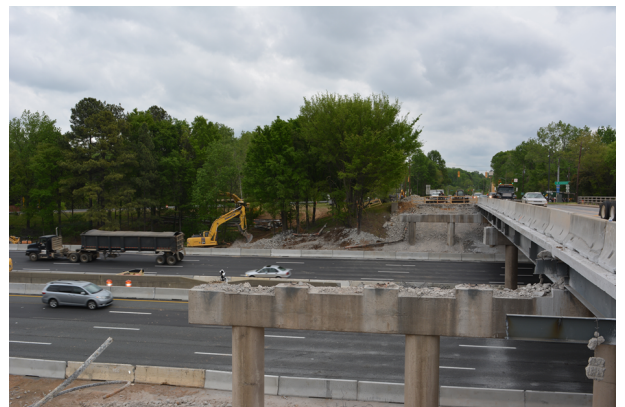
Demolition of the northern half of the LaSalle Street bridge
