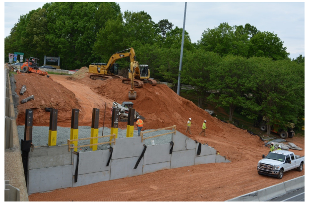
MSE (mechanically stabilized) wall construction at Griffith Street bridge
