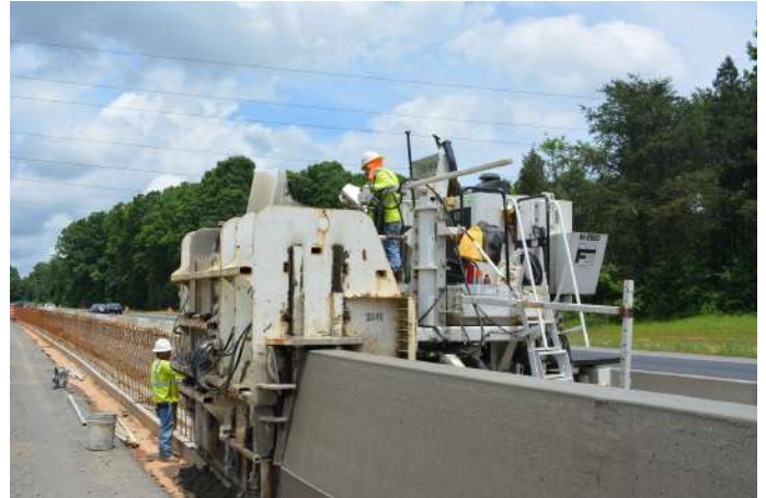
Constructing permanent concrete barrier in Mooresville
