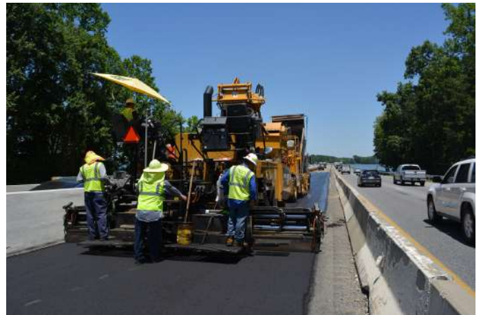
Paving the causeway near the Griffith Street bridge in Davidson
