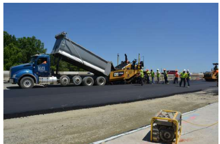
Paving northbound I-77 near the I-77/I-85 interchange
