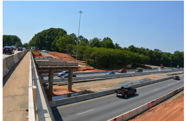
Construction of the new Griffith Street bridge in Davidson
