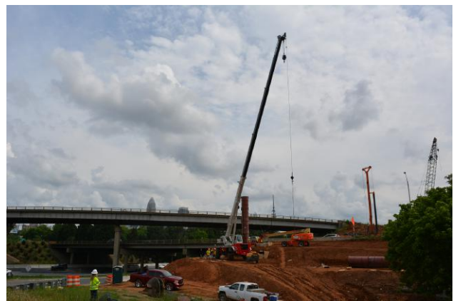
Forming columns at the new bridge from I-277 westbound to I-77 southbound in Charlotte
