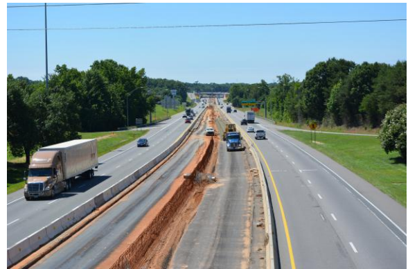
Soil stabilization activities near Exit 35 in Mooresville
