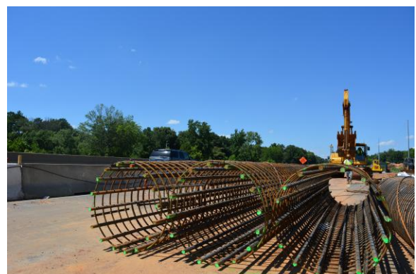
Rebar cages for the foundation of the new Oaklawn Avenue bridge
