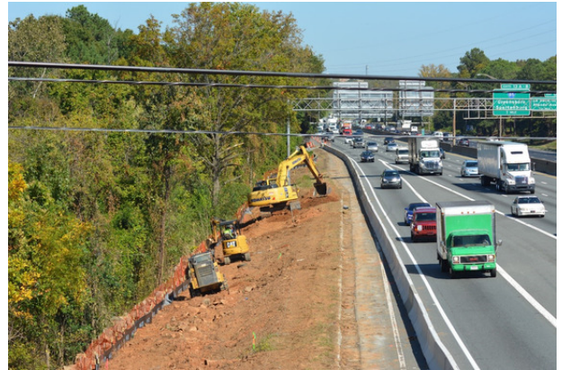
Clearing operations in the south segment by the I-77/Brookshire Fwy. interchange
