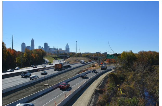
Preparing the area for the upcoming traffic shifts near uptown Charlotte
