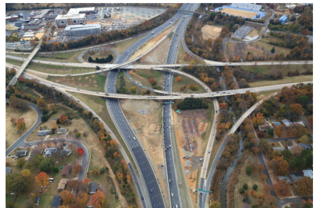
Construction activities near uptown Charlotte
