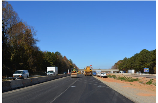
Paving operations in north segment
