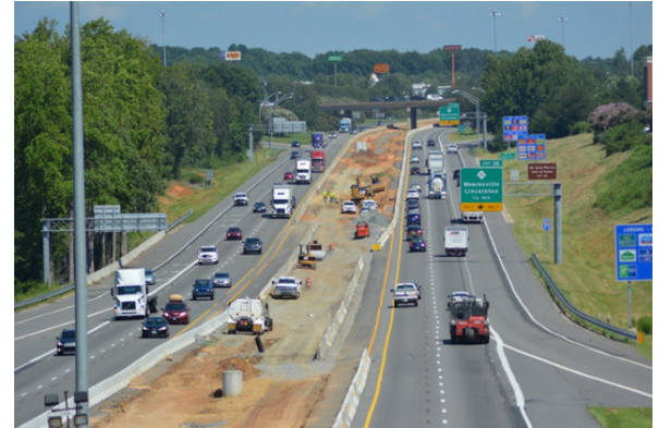
Grading operation south of Exit 36 (Plaza Dr.)
