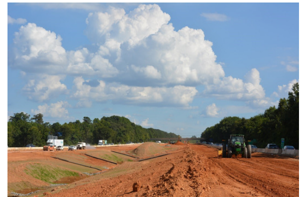
Grading activities south of Exit 25 (Sam Furr Rd.)
