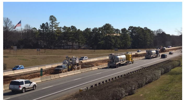
Permanent concrete barrier work near Exit 28 (Catawba Ave) near Cornelius
