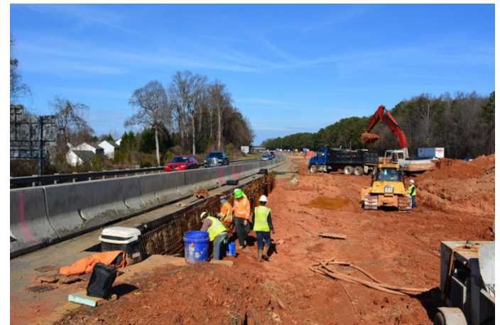
Pedestrian culvert work near Huntersville
