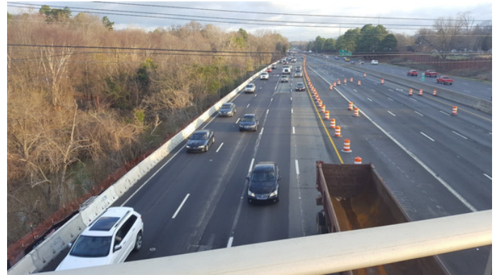
Traffic shift on I-77 near uptown Charlotte
