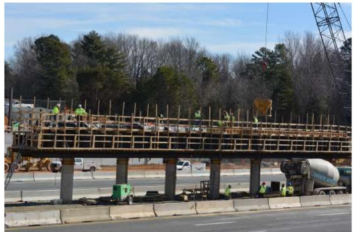
Construction crews working on column caps at the new Hambright Road direct connector bridge in Huntersville.
